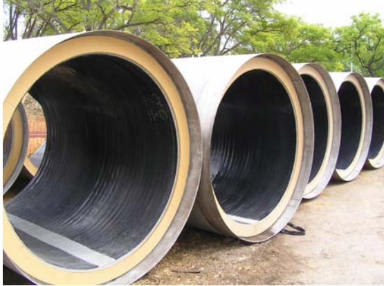
Figure 1 - Jacking Pipes with Stainless Steel Collars & Thermoplastic Lining
